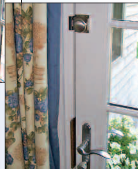
Concealed Door Closure - latch at 54" for child safety.
