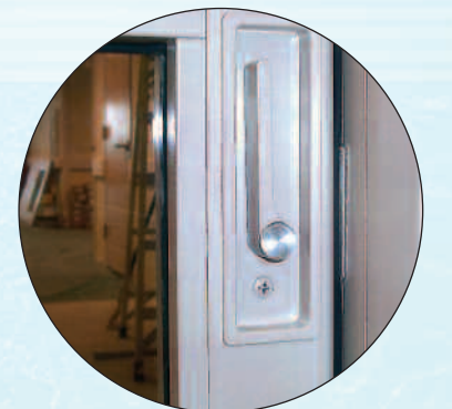
Recessed handle prevents patient/equipment hang-ups, when moving through doorway
