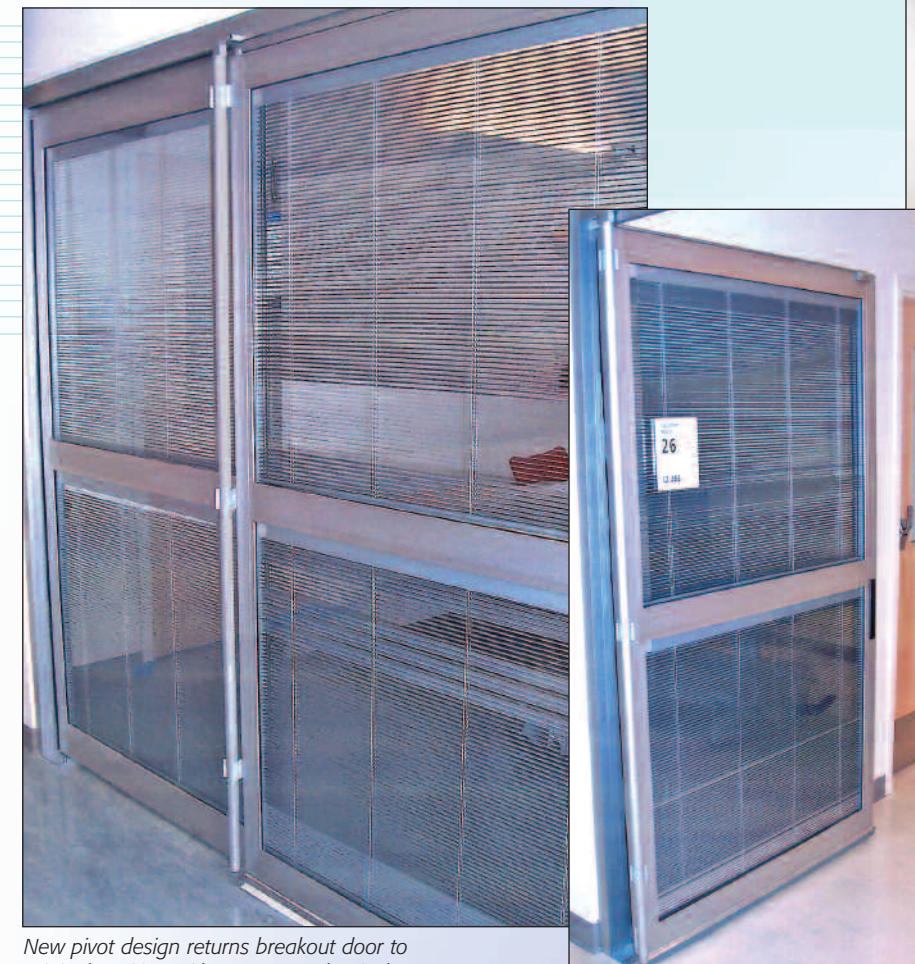
Sliding door in breakout position
